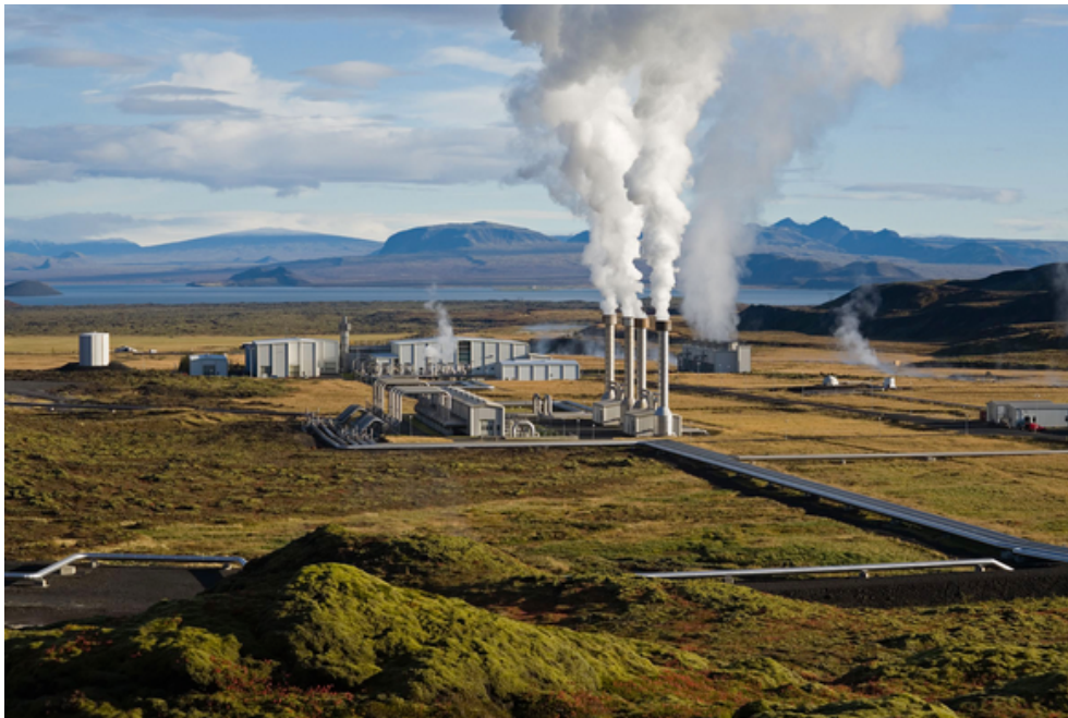
Figure 2: Nesjavellir power plant
